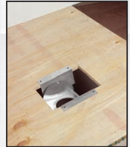
Mount SureGrip support plate.
