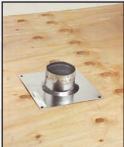
Push pipe through vent support.
